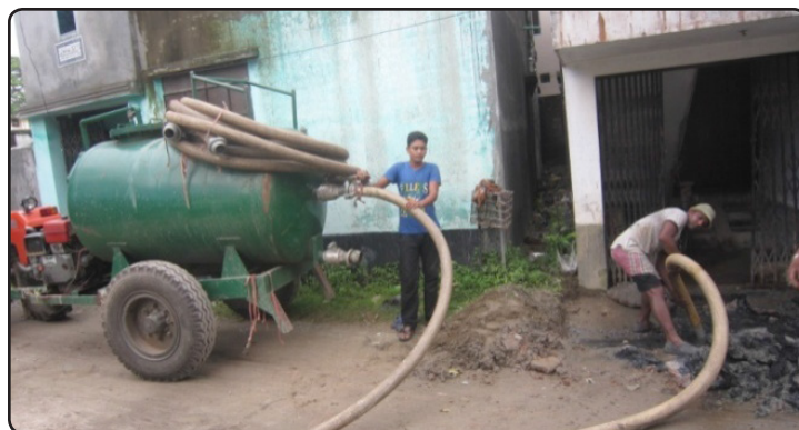
Mechanical emptying of septic tanks/pits using 'vacutugs' needs to be encouraged.
