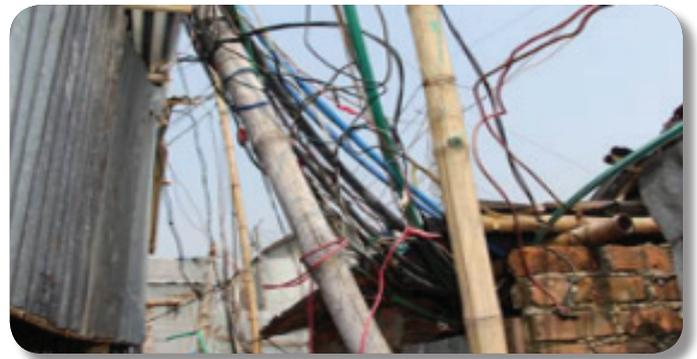
Figure 3: Unsafe electricity lines at Mohakhali slum; this often causes accidents and fire outbreaks.
